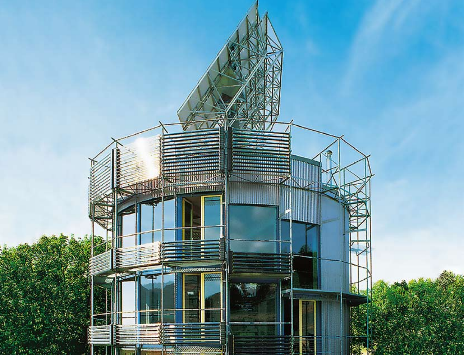
Example for use of Vitosol tube collectors on a wall.
